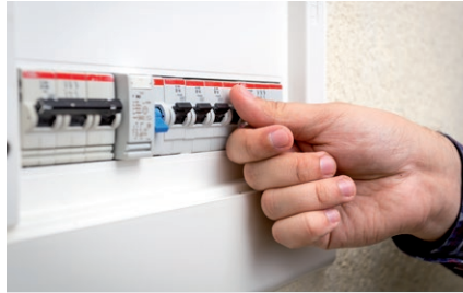
EICR (Fixed Wire Testing)
