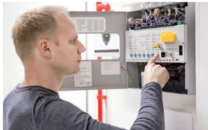
Fire Alarm Testing and Servicing
